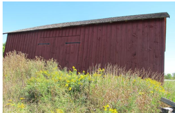
Figure 15 Dickerson Barn, west elevation
