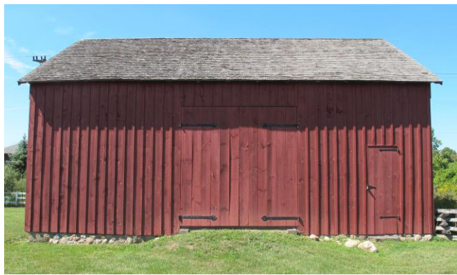
Figure 13 Dickerson Barn, east elevation
